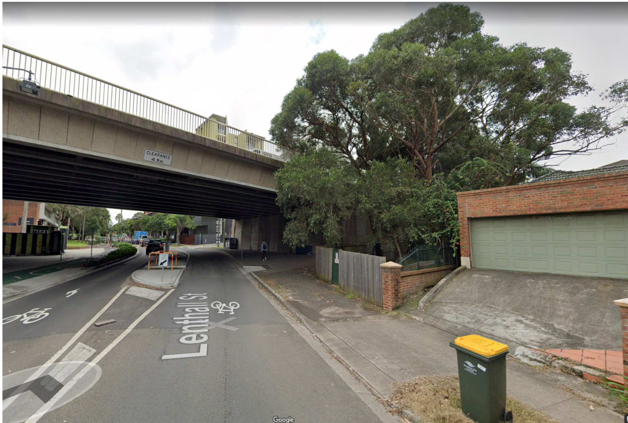
b) View of Bridge over Lenthall St
